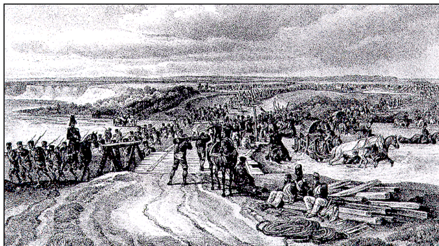
Crossing the Dniepr – August 11, 1812. In this lithography we see the columns of infantry and their supplies crossing the river. In the middle, the French engineers are building a bridge with trestles.
